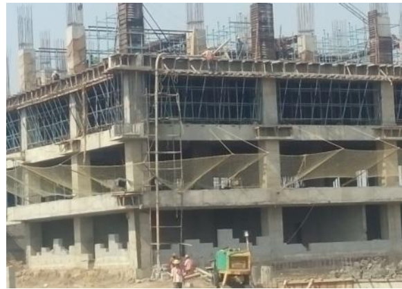
SPV Building 4 th floor column progress
