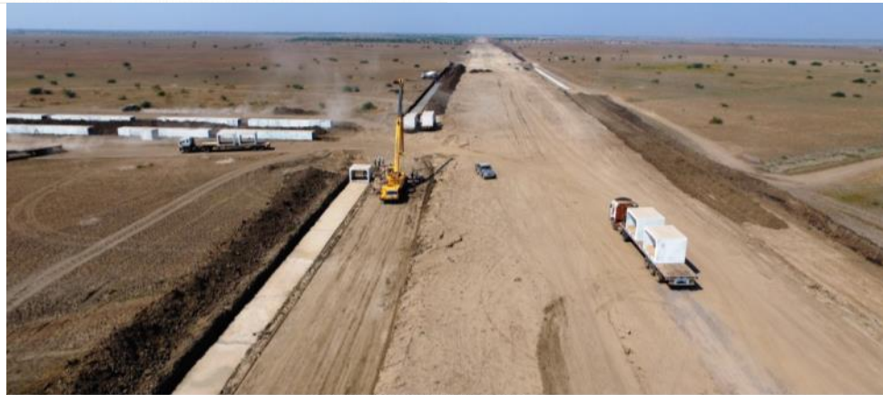
Power Duct Laying In Progress. - H-1
