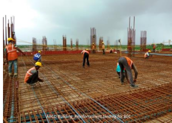
Reinforcement for BEC Slab
