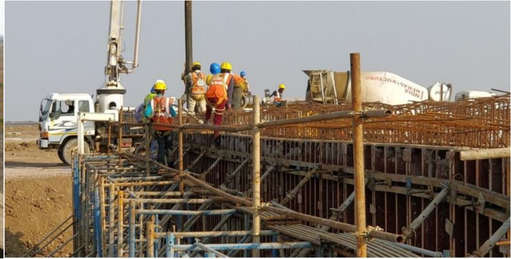
E-3 BRIDGE: SUBSTRUCTURE CONCRETING
