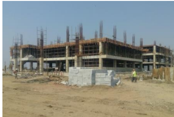
BEC 2 nd Slab Shuttering
